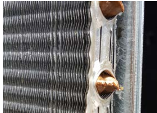
« A close up, side view of the fins of a very common condenser coil.
